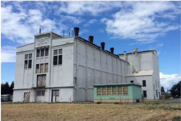
Georgetown Steam Plant—Seattle, WA
